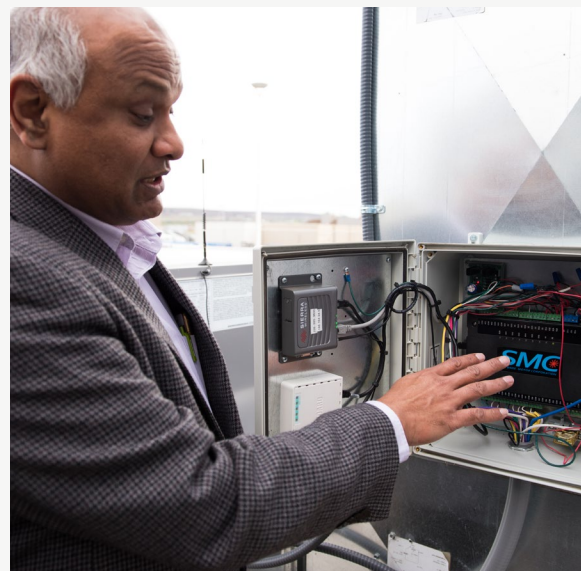
An engineer studies an advanced building control system that reduces energy use in building operations. Photo: Andrea Starr | Pacific Northwest National Laboratory.
